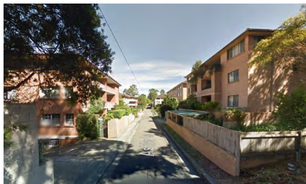
PICTURE 6 – ASHLEY LANE RESIDENTIAL TO WEST OF RSL CLUB AND CAR PARK
