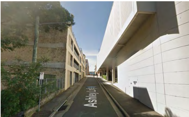
PICTURE 3 – ASHLEY LANE BETWEEN CLUB AND CAR PARK
